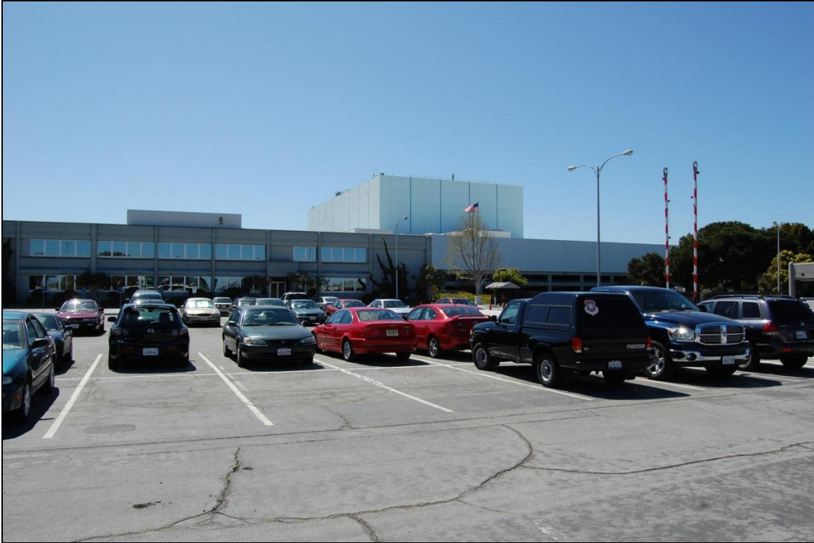
Photo 3: View looking southeast toward Building 1002 (left), Building 10031 (right), and Building 1003 (rear).
