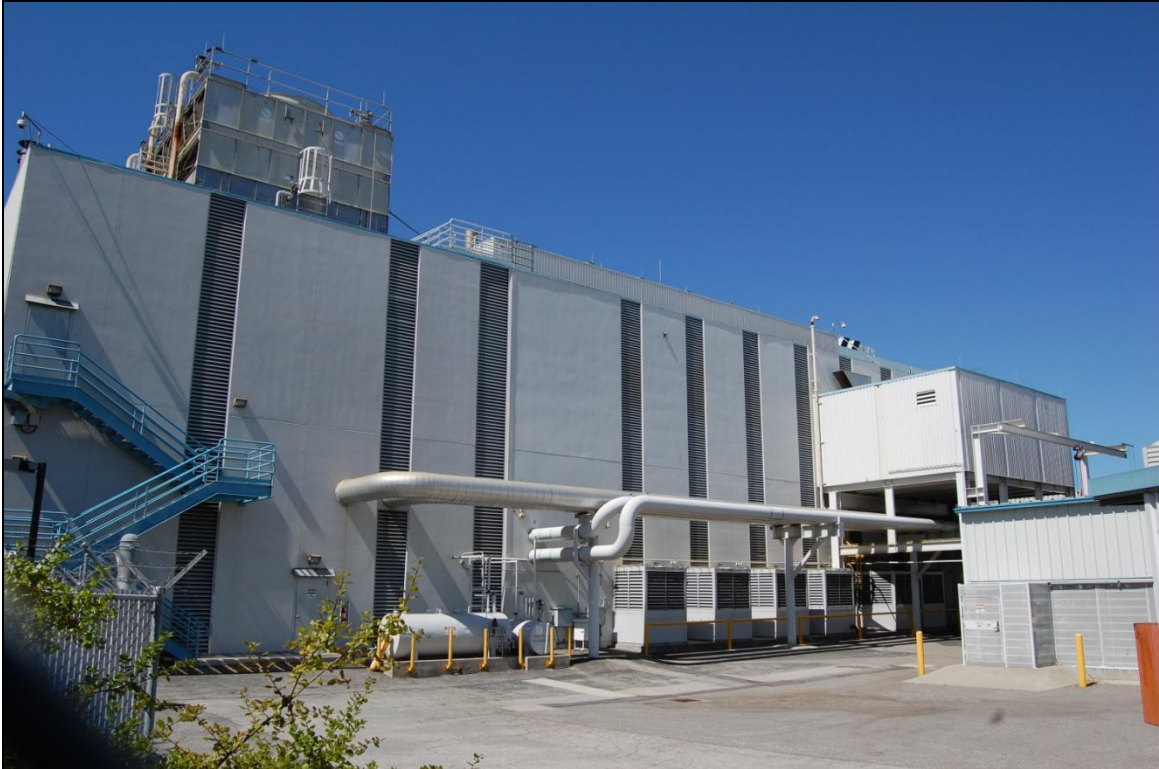
Photo 6: View looking west toward Building 1004.
