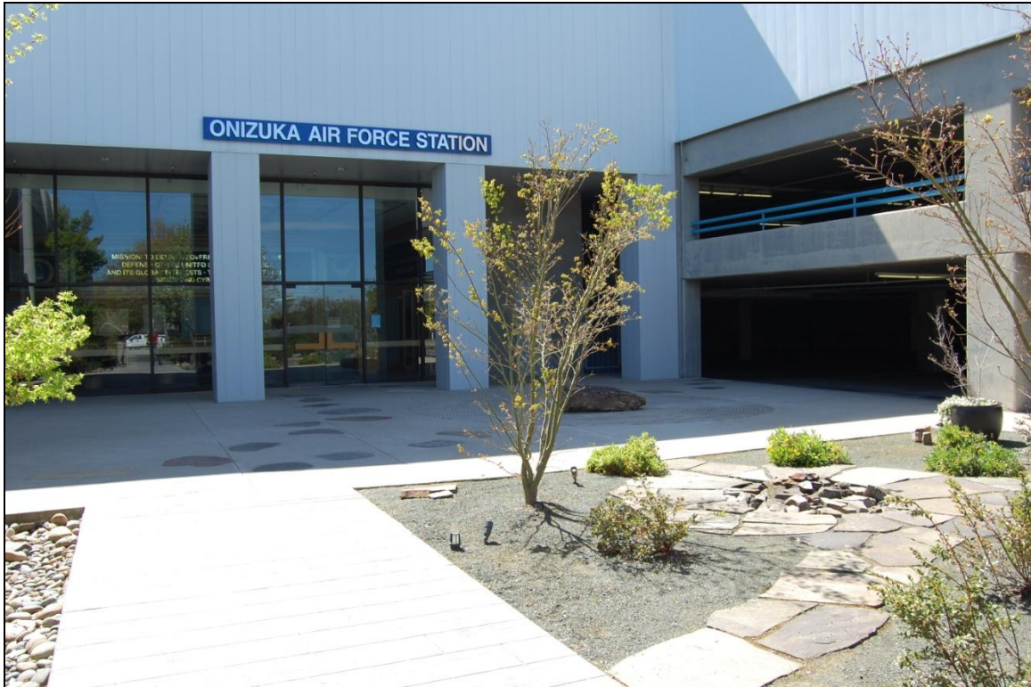
Photo 1: View looking south toward entrance to Building 10031. This entrance provides access to Buildings 1001, 1002, 1003, 1004, and 10032 because all buildings are interconnected.
