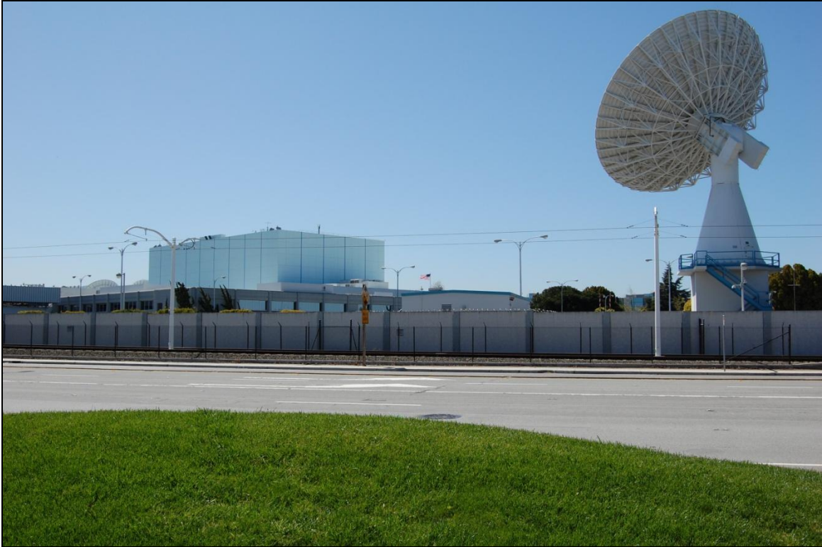
Photo 5: View looking southeast toward Building 1002 (foreground) and Building 1003 (background).
