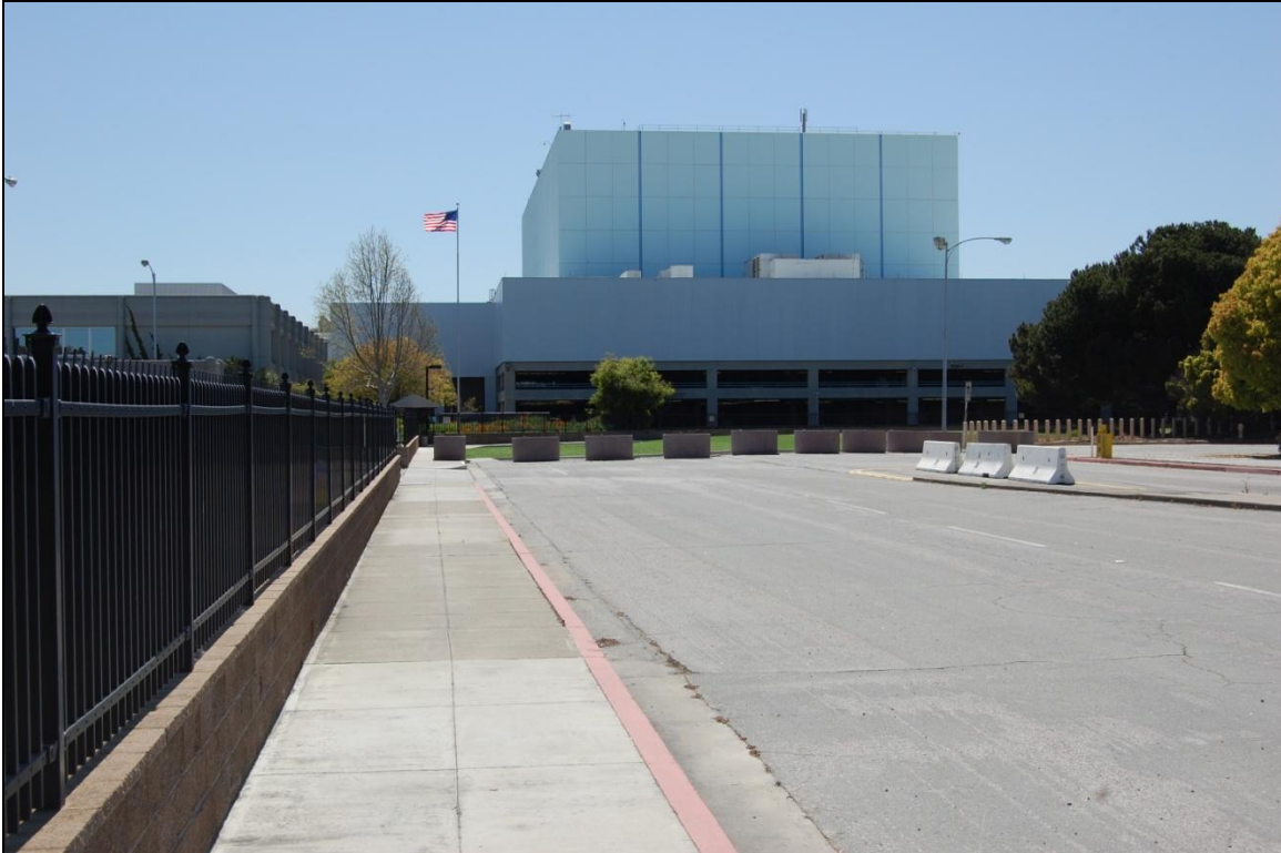
Photo 4: View looking south toward Building 10031 (foreground) and Building 1003 (background).
